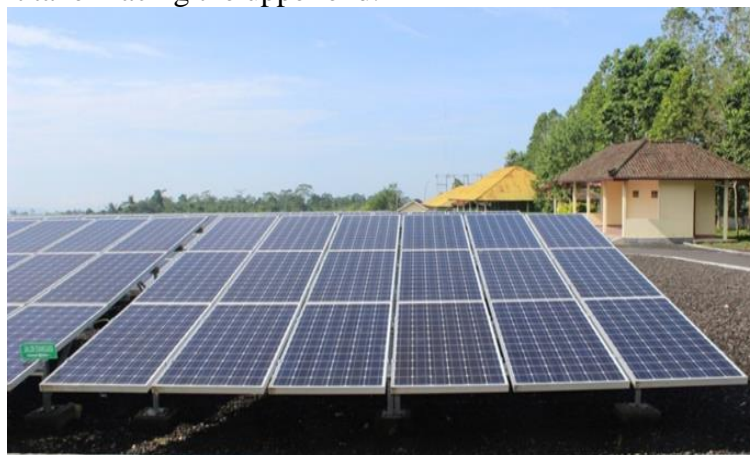
Figure 24 Array installation of 1 MW Kayubih PV plant
